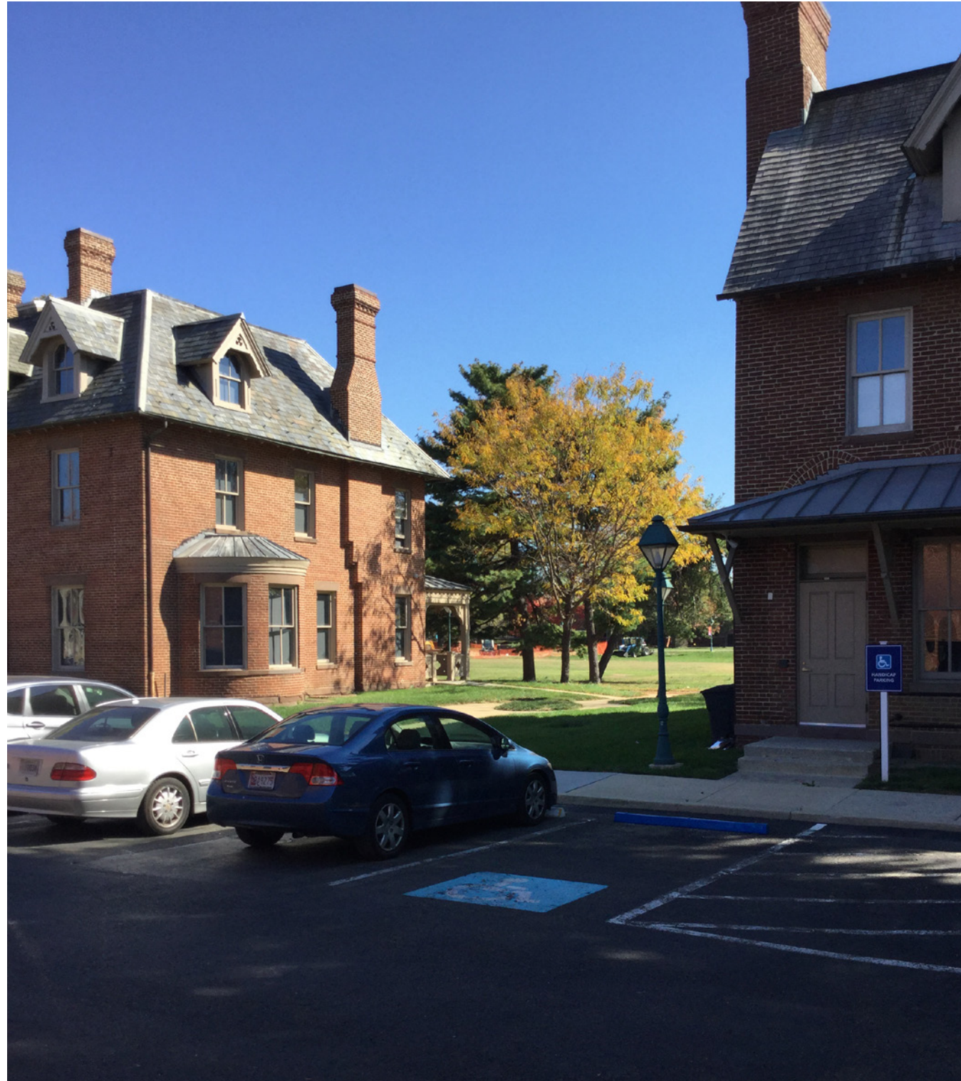
9. Rear view of Fay and Ballard House and Olmsted Green beyond
